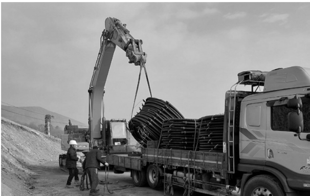
Fig. 5. View of strand anchors rolled in bundles
